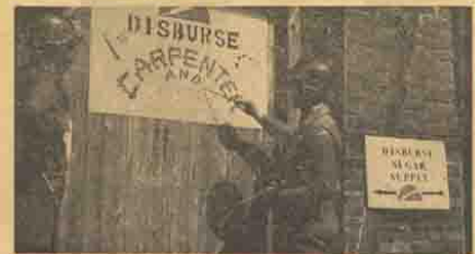
CARPENTER and Sign Shop gets finishing touches by Pfc. Howard Romnich of "A" company who is at present attached to Service. Looking on is most-trust regimental carpenter T/S Vernon Peters.
